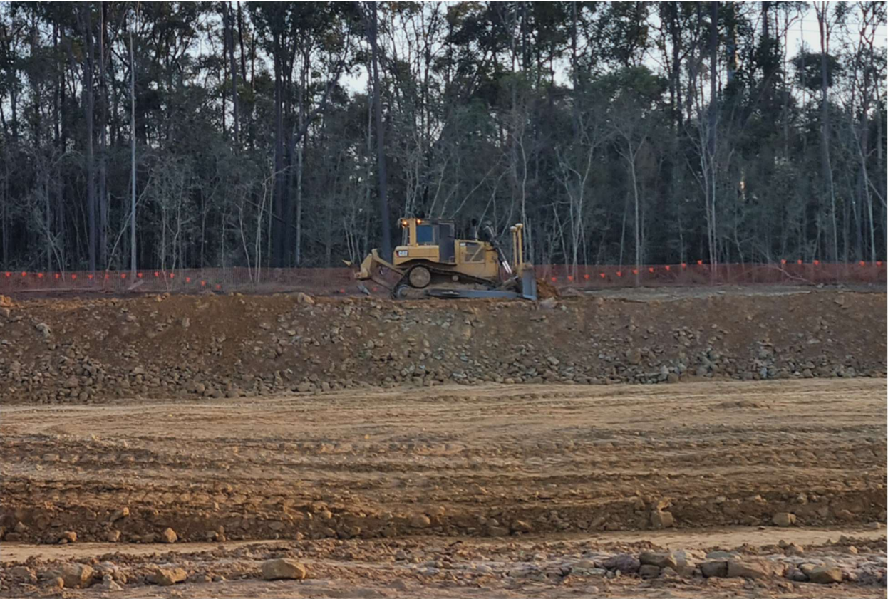
Figure 4: View of the Site during construction
