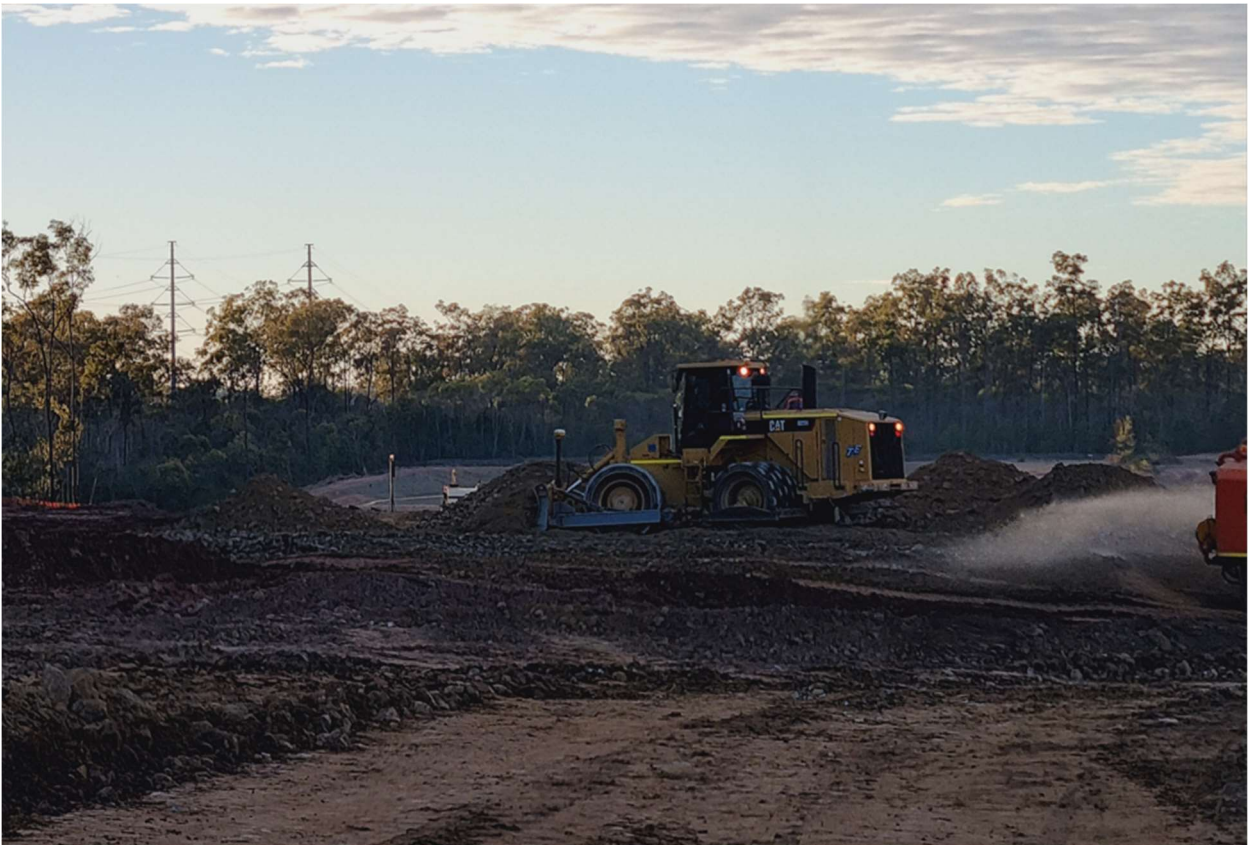
Figure 3: View of the Site during construction
