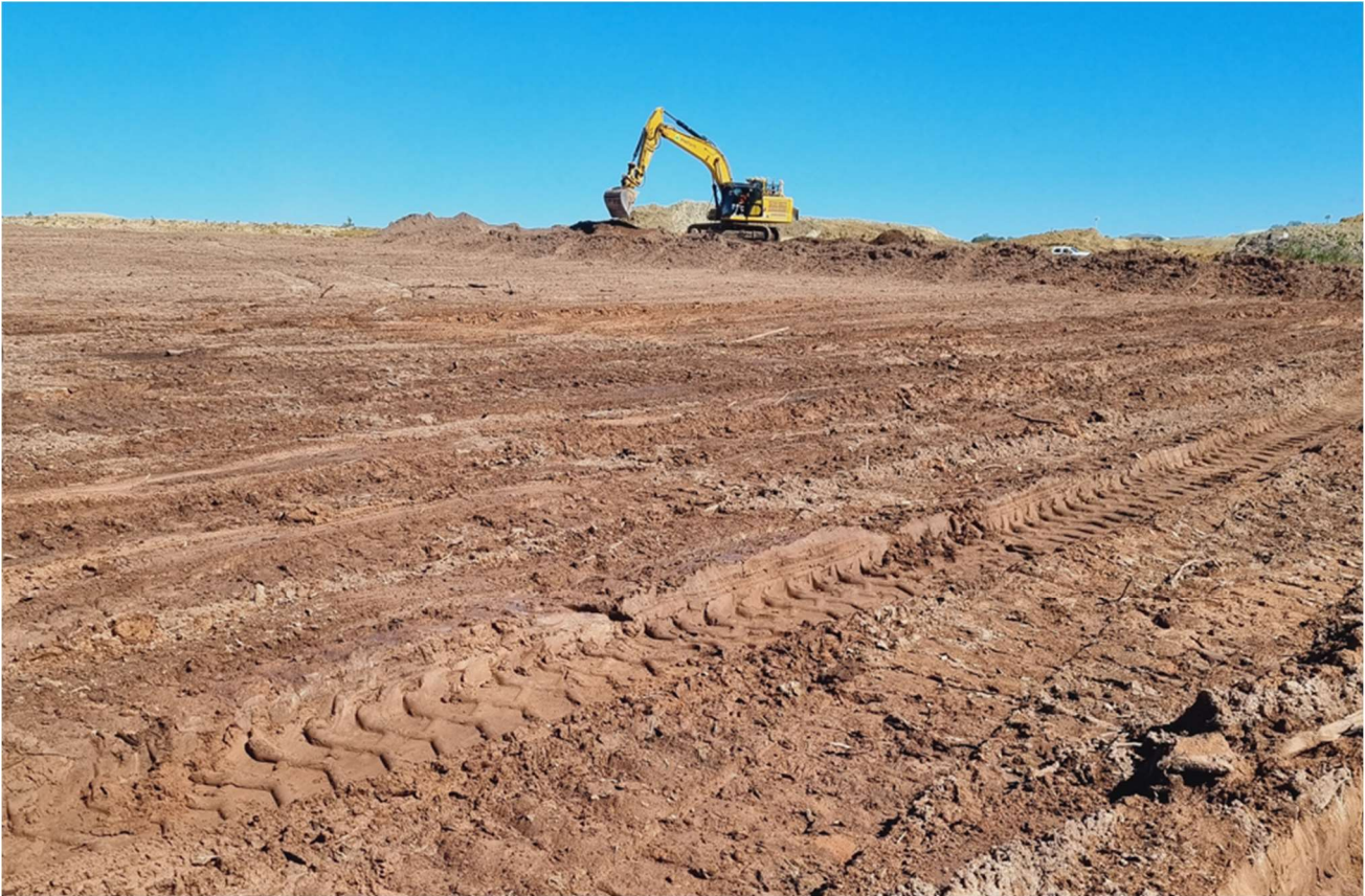
Figure 2: View of the Site during Stripping Operations
