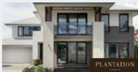
MAJESTIC - CONTEMPORARY FAÇADE
