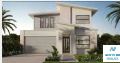
THE ASPEN - FORESHORE FAÇADE
