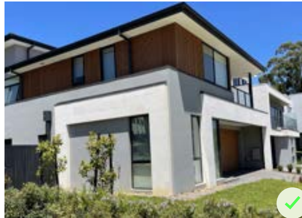
Continuation of materials used on the primary street facade returns to the side of the home minimum 3m.
