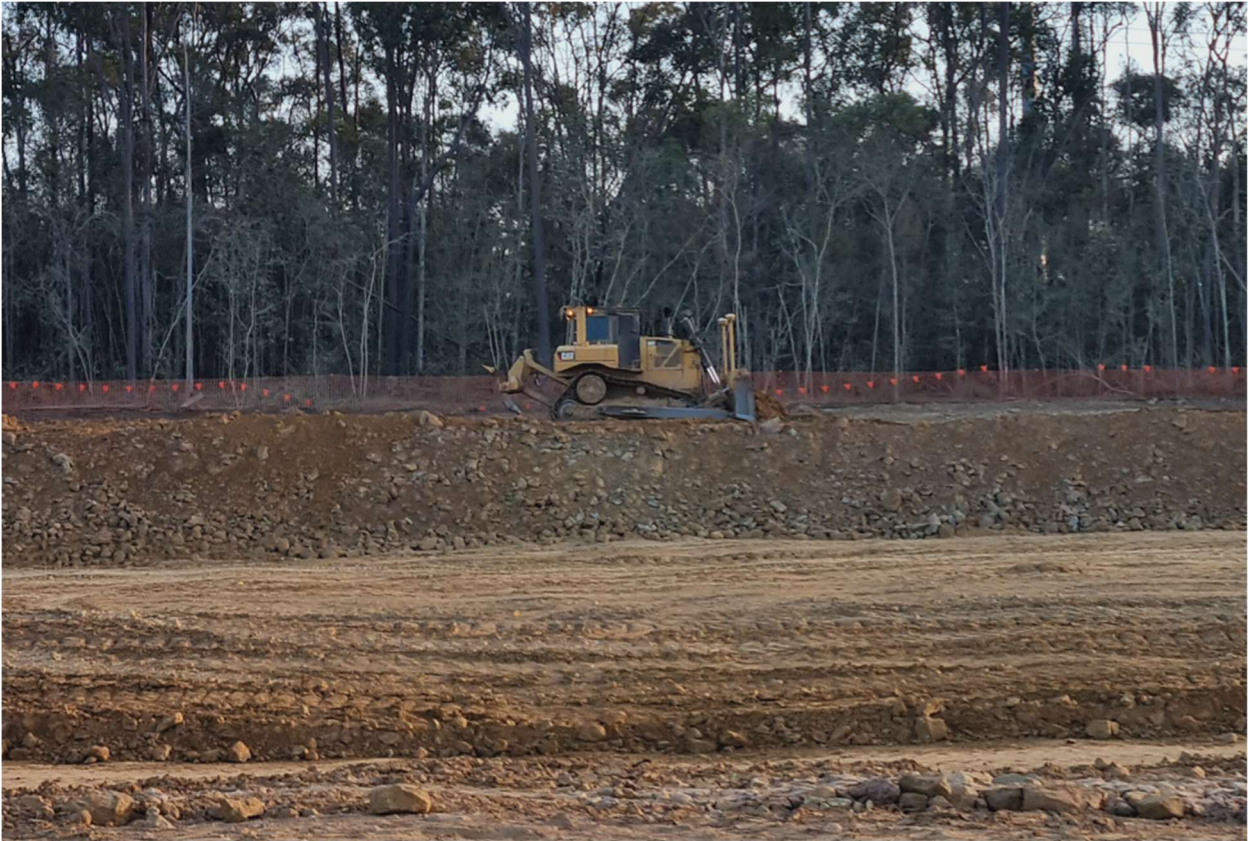
Figure 4: View of the Site during construction
