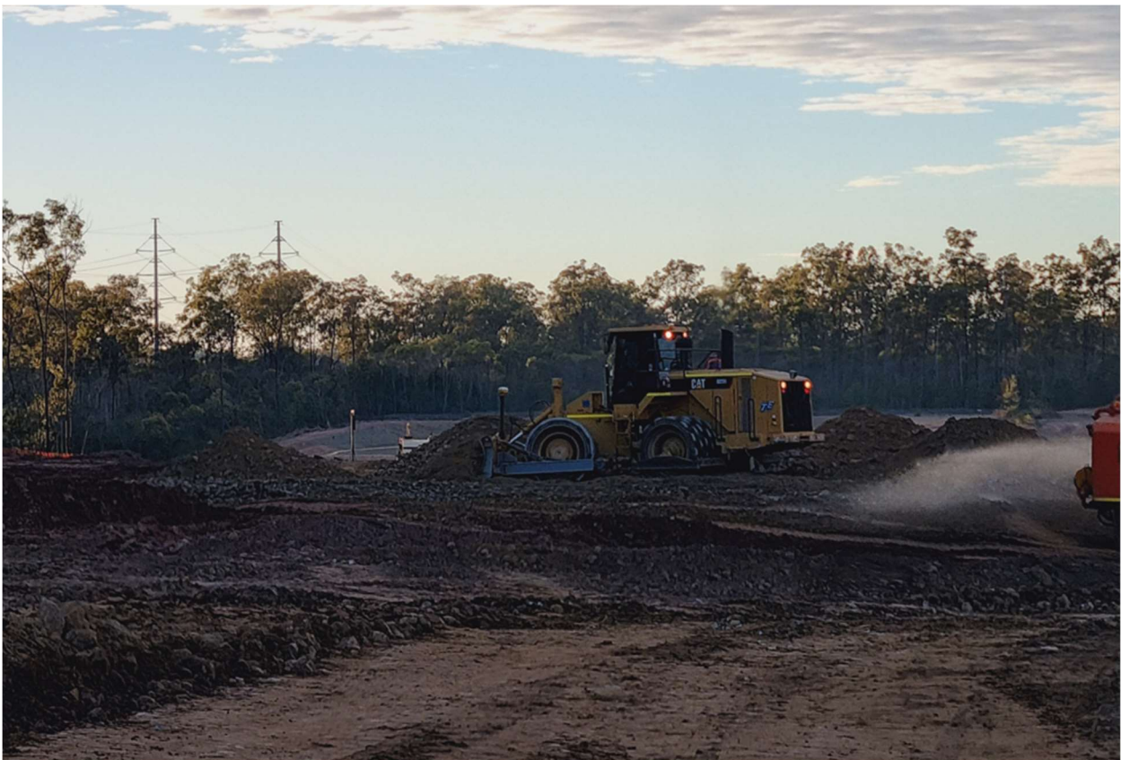
Figure 3: View of the Site during construction
