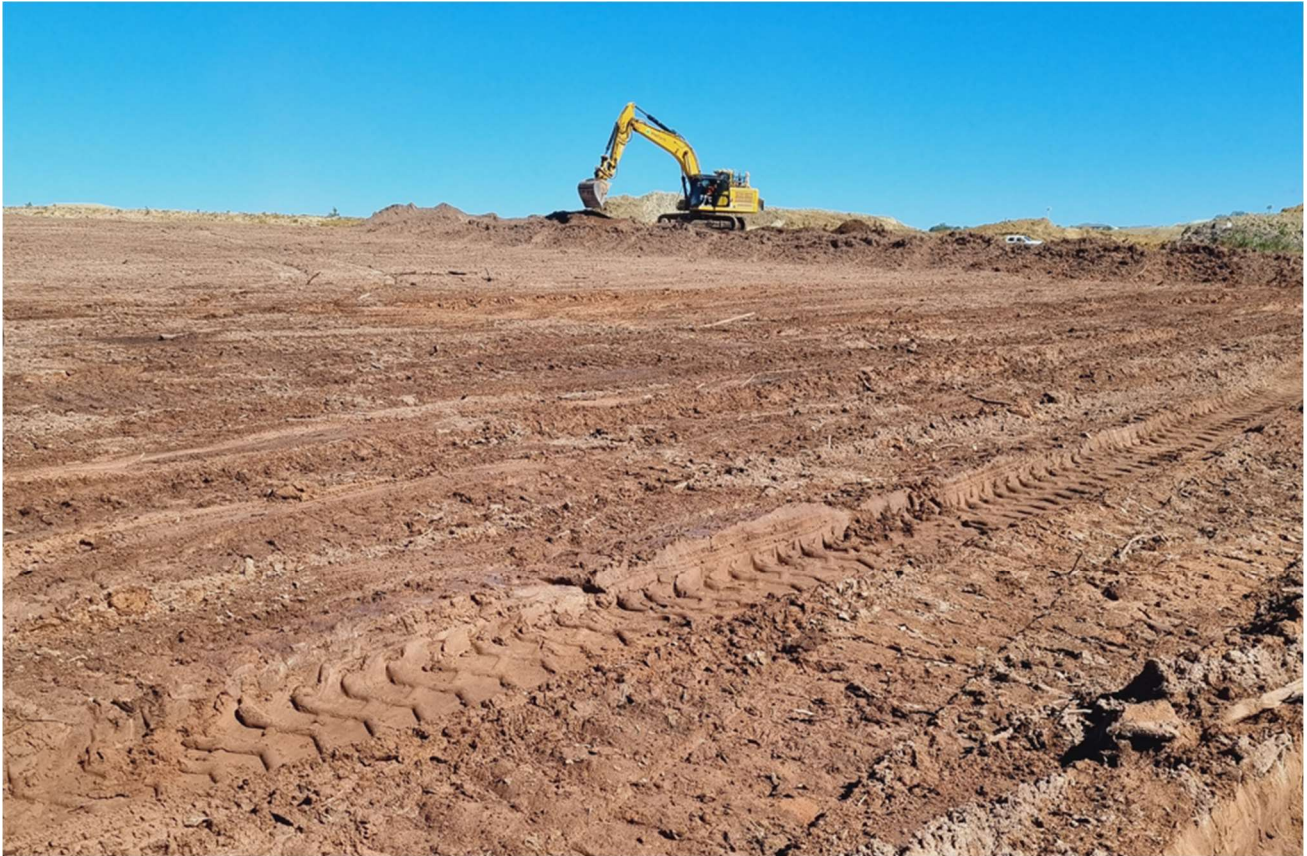
Figure 2: View of the Site during Stripping Operations
