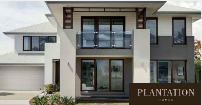
MAJESTIC - CONTEMPORARY FAÇADE
