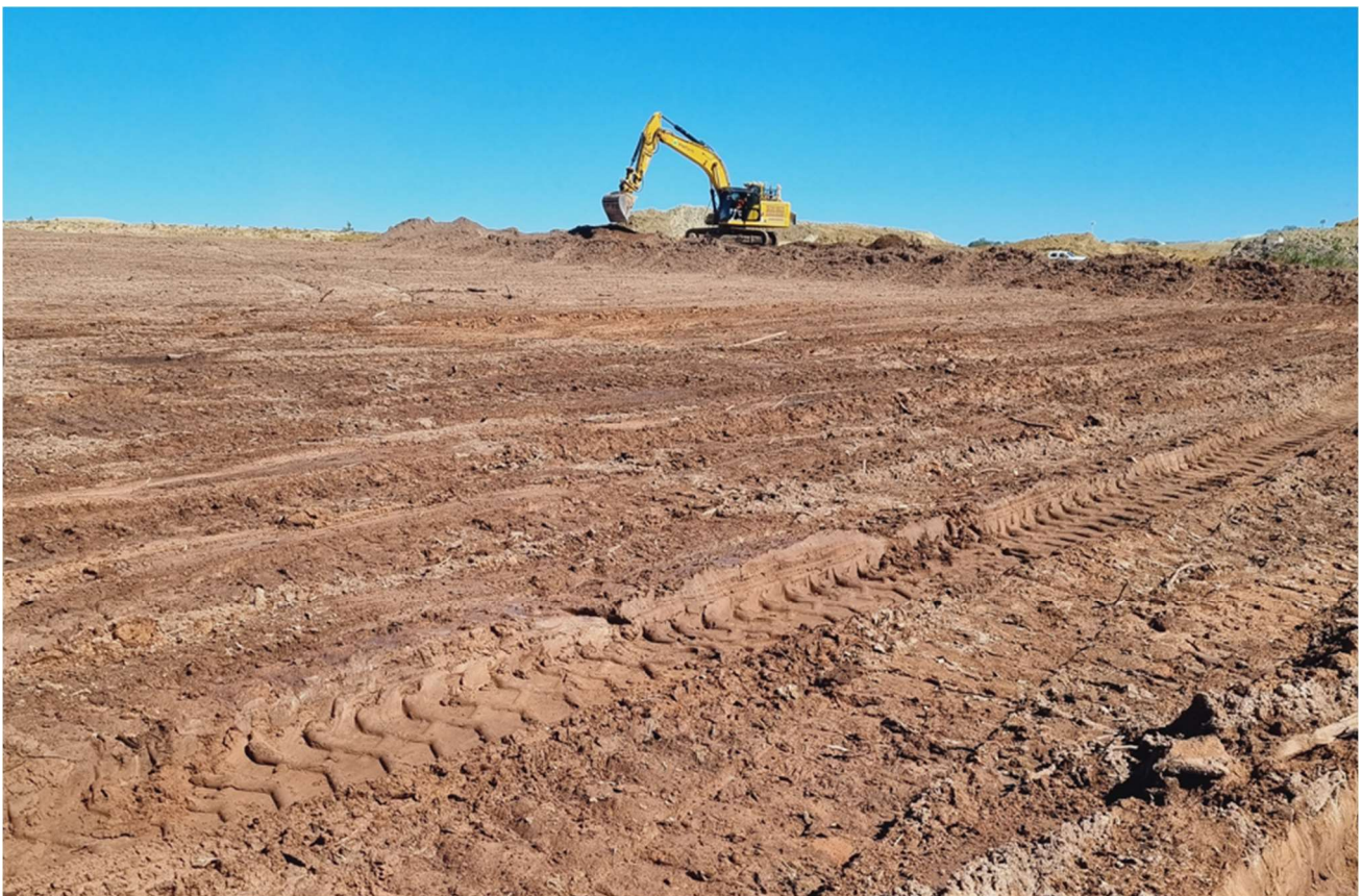
Figure 5: View of the Site during Stripping Operations
