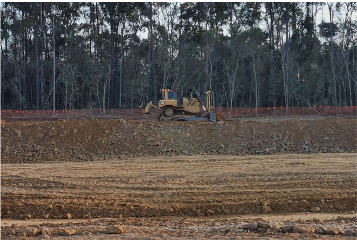
Figure 7: View of the Site during construction
