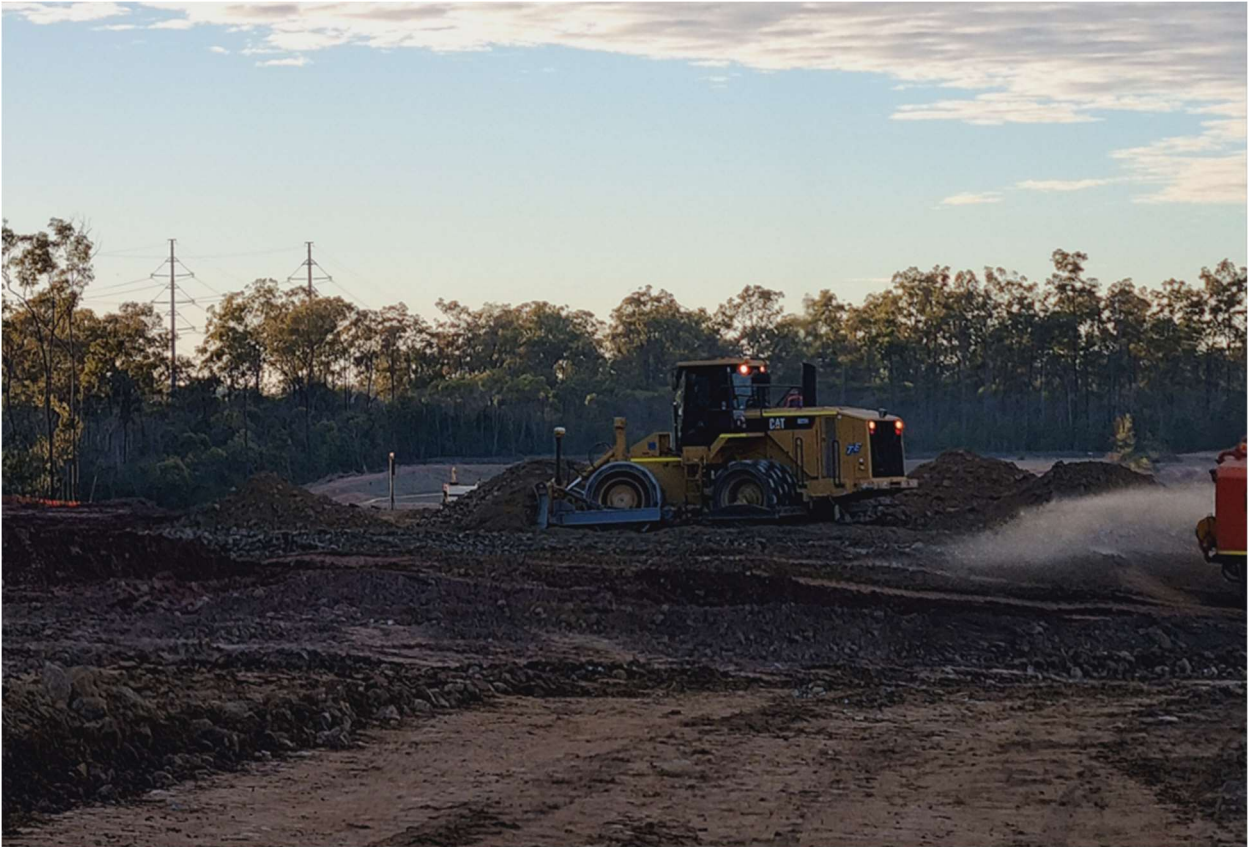
Figure 6: View of the Site during construction
