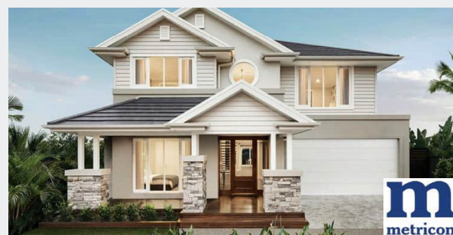
THE BAYVILLE - 49A FACADE
