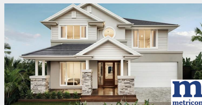
THE BAYVILLE - 49A FAÇADE
