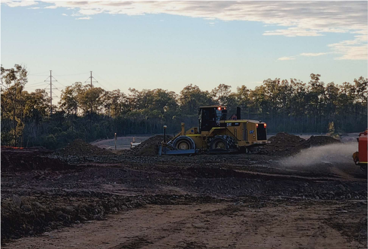
Figure 6: View of the Site during construction
