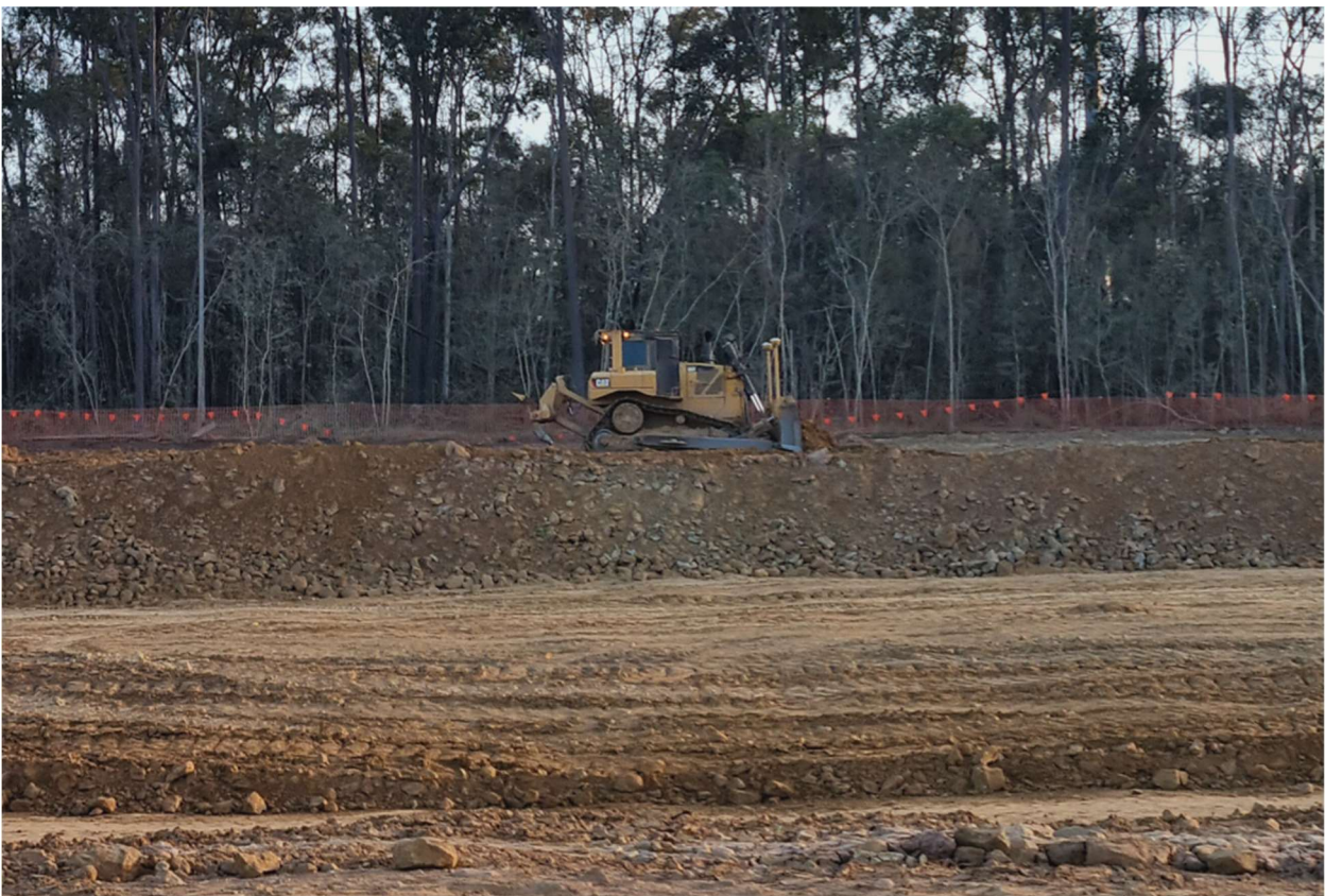
Figure 7: View of the Site during construction
