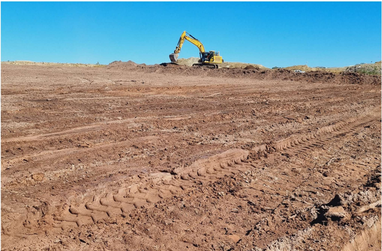
Figure 5: View of the Site during Stripping Operations
