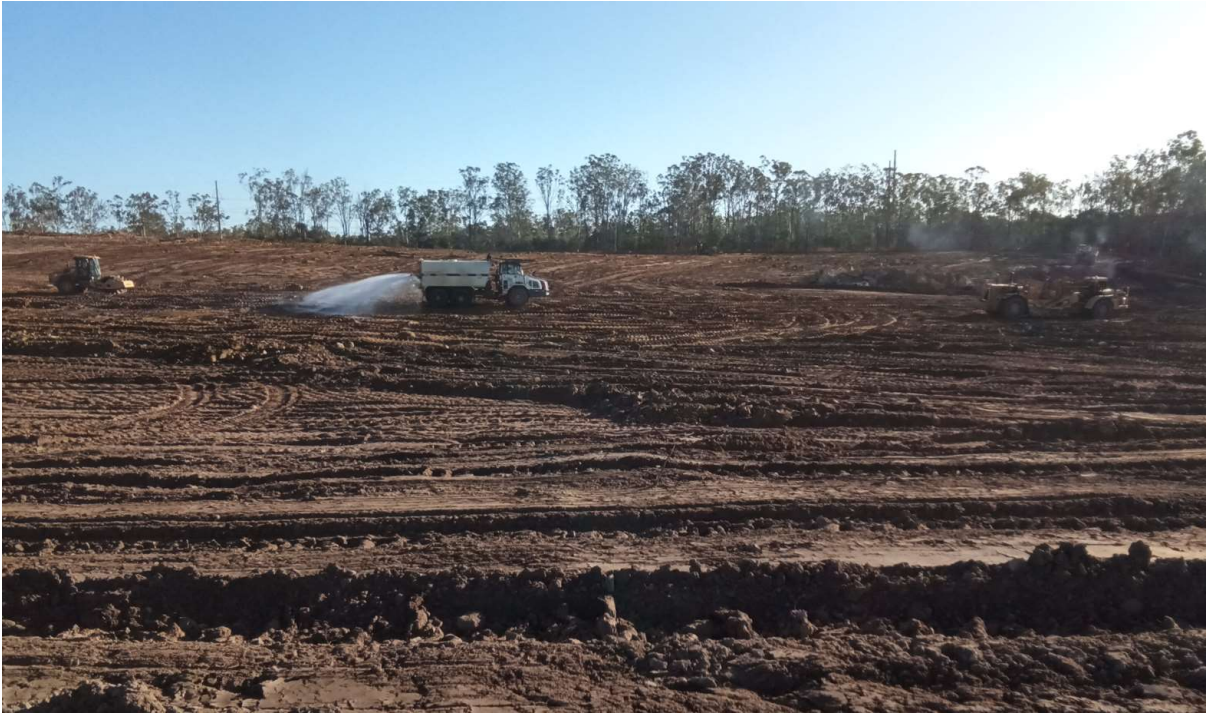
Picture 3: View of the Site During Construction
