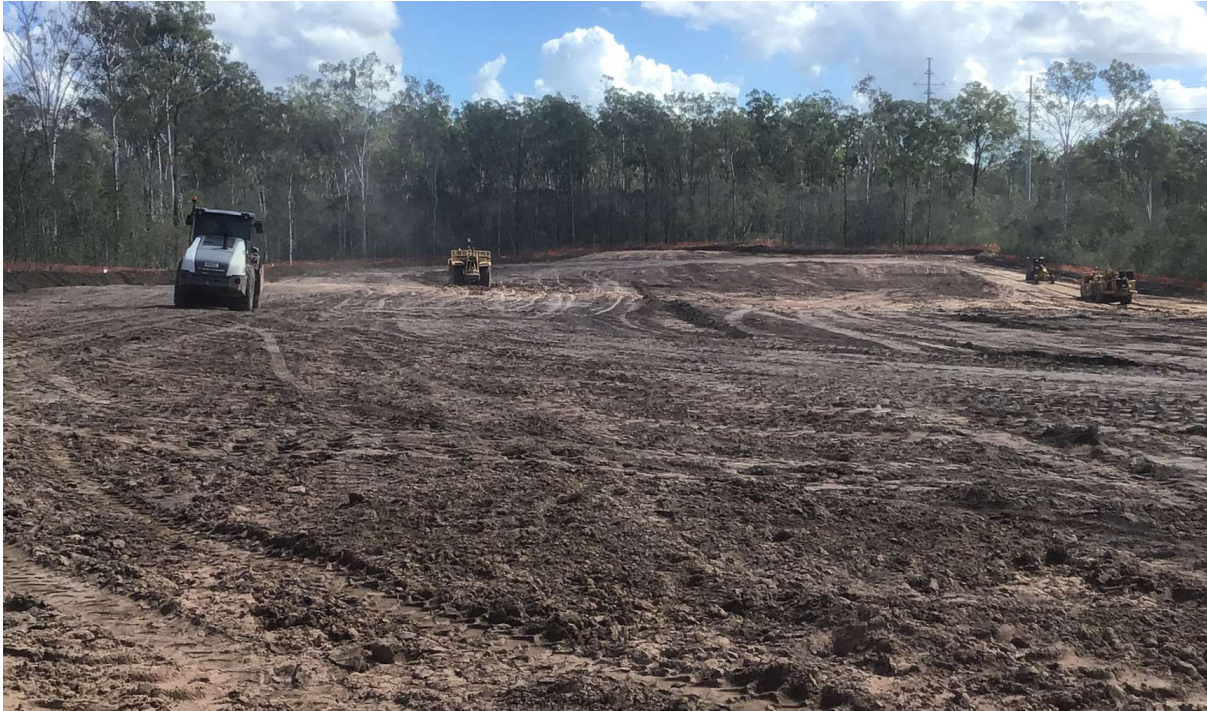
Picture 1: View of The Site During Stripping Operations
