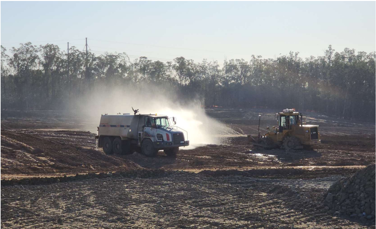
Picture 4: View of the Site During Construction
