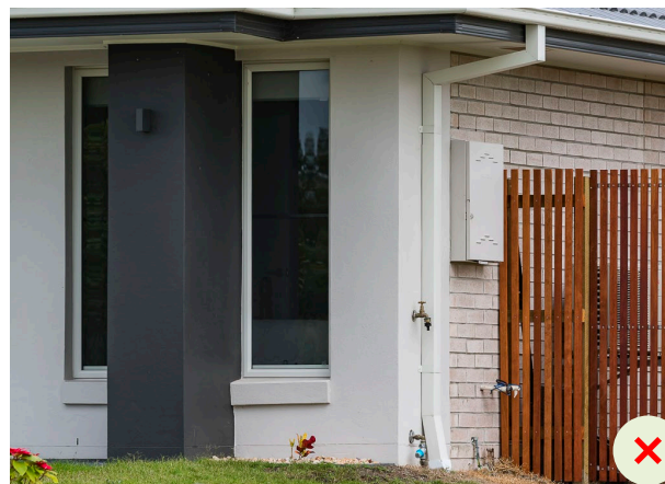
Render not returned minimum 3m from front facade
