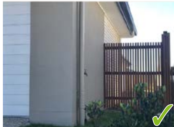
Render or material finish must return back around the walls at least 1m or wherever the side fence meets the house
