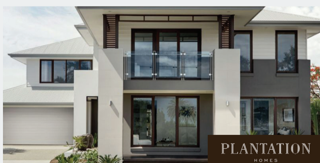
MAJESTIC - CONTEMPORARY FAÇADE
