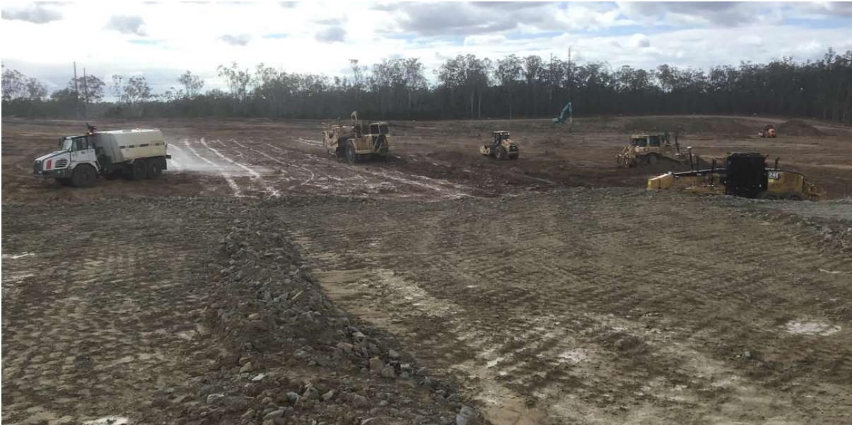
Picture 4: View of the Site During Construction
