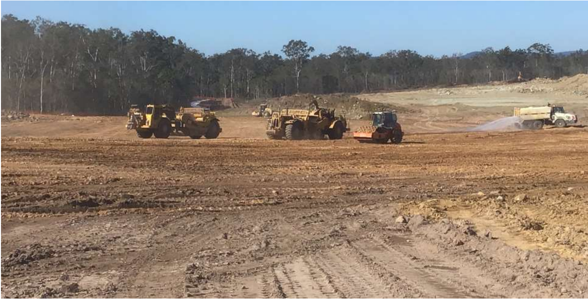
Picture 3: View of the Site During Construction
