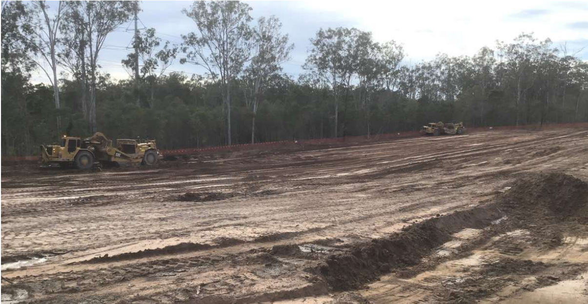
Picture 1: View of The Site During Stripping Operations
