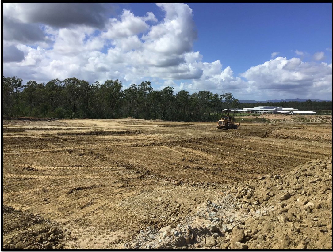
Picture 3: View of the Site During Construction
