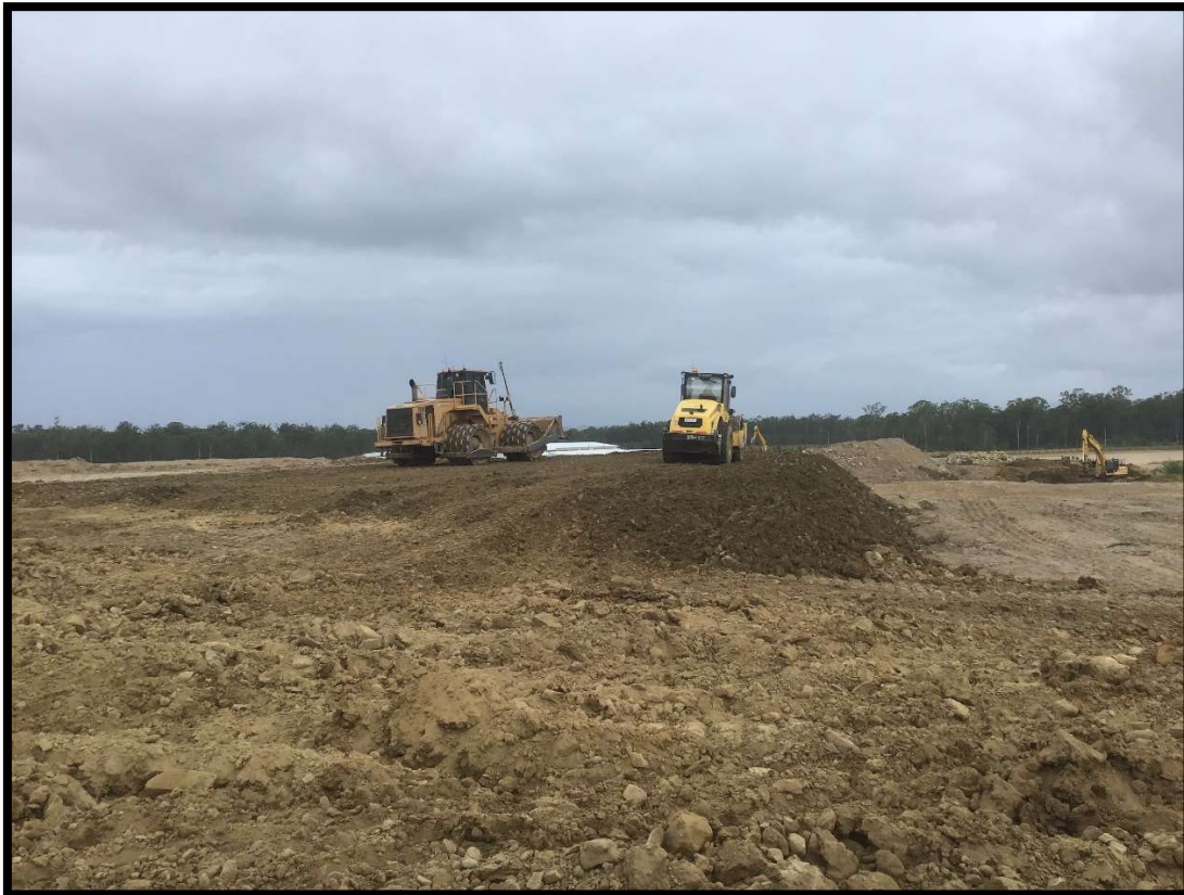
Picture 4: View of the Site During Construction
