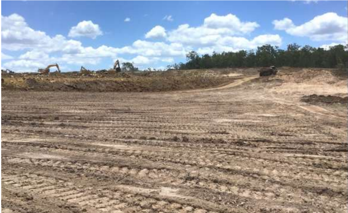
Picture 1: View of The Site During Stripping Operations
