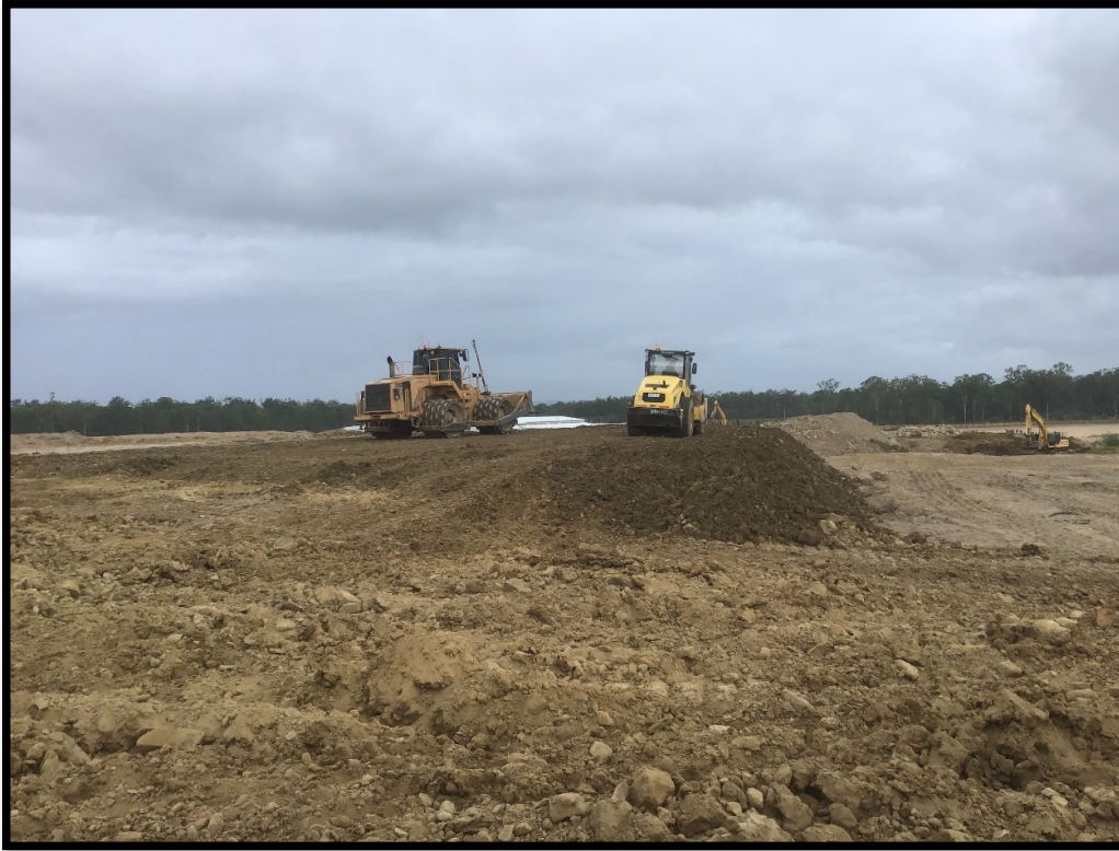
Picture 4: View of the Site During Construction
