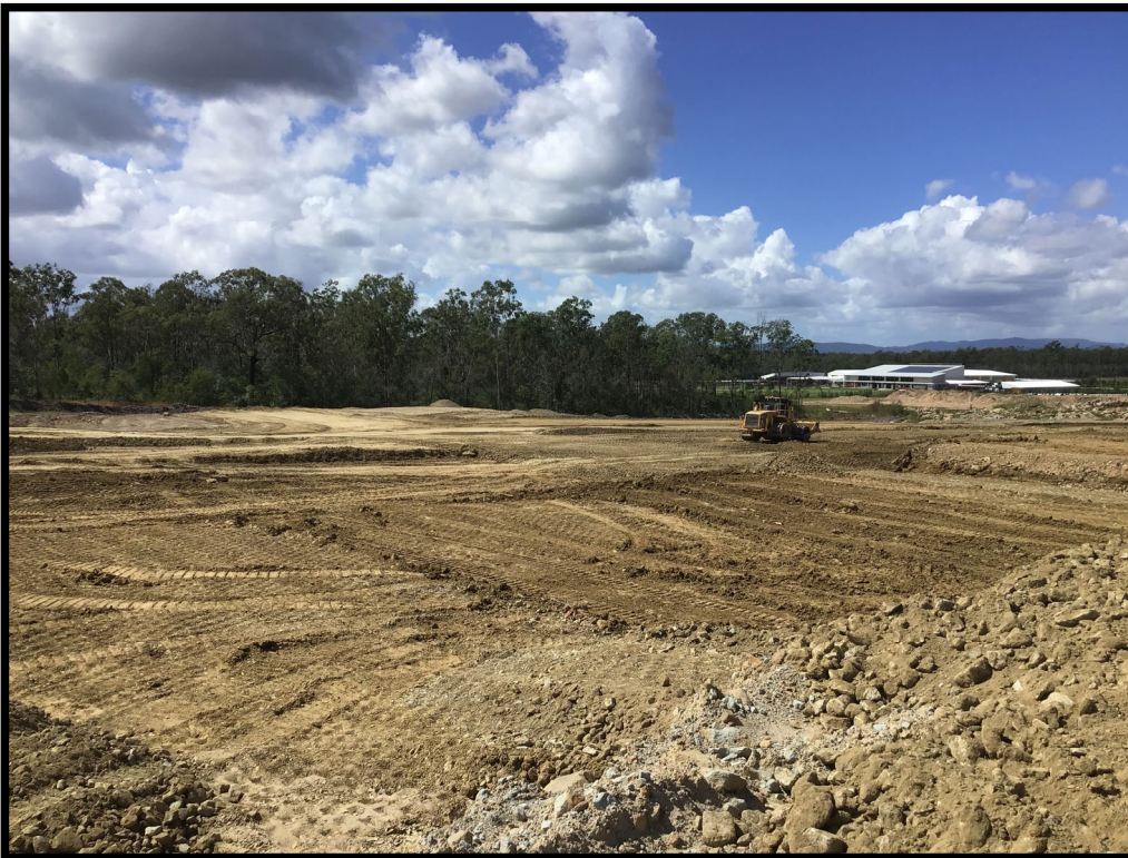
Picture 3: View of the Site During Construction
