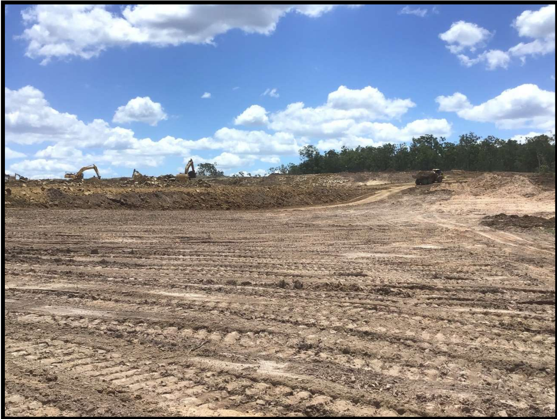
Picture 1: View of The Site During Stripping Operations
