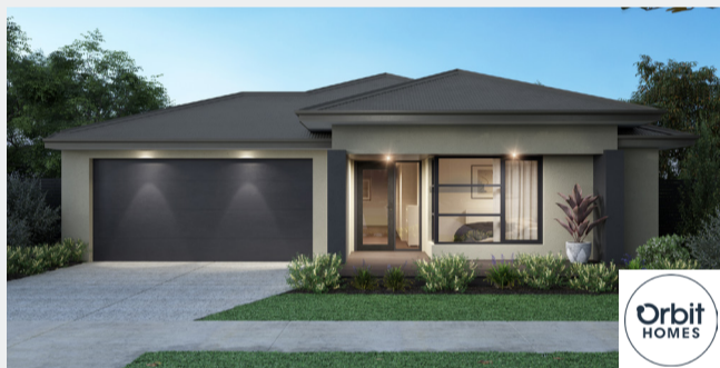
THE CAULFIELD - MADRID FAÇADE
