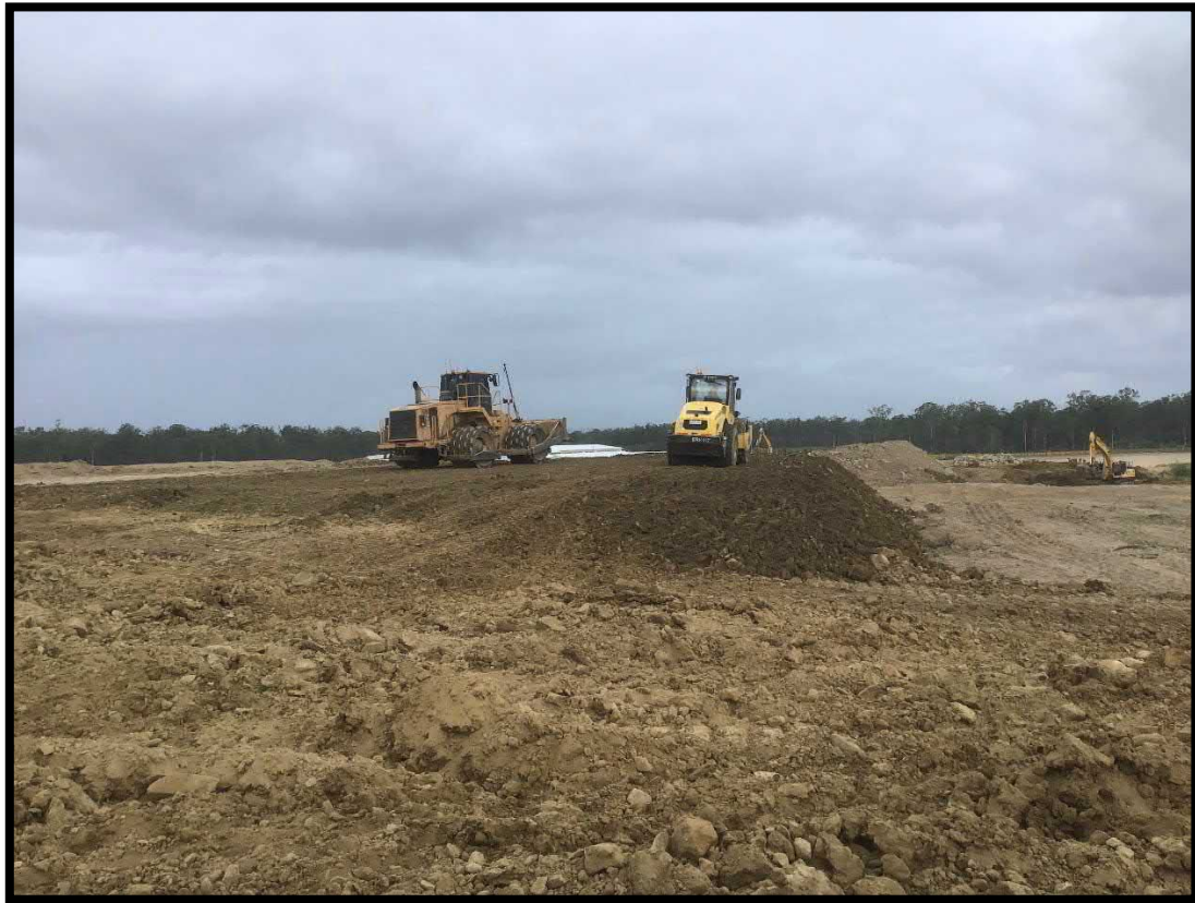
Picture 4: View of the Site During Construction
