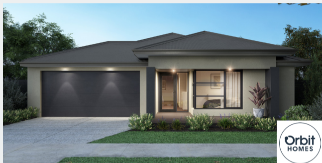
THE CAULFIELD - MADRID FAÇADE
