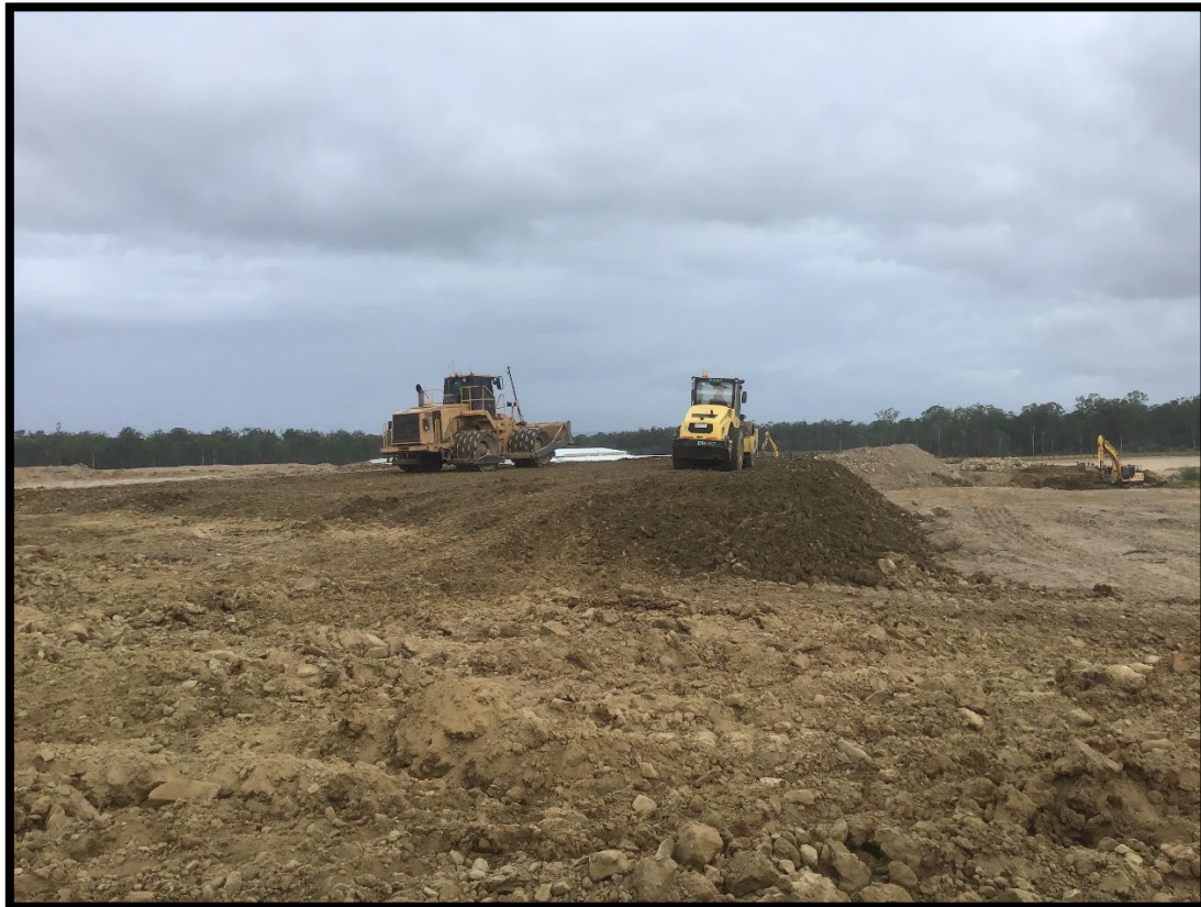
Picture 4: View of the Site During Construction
