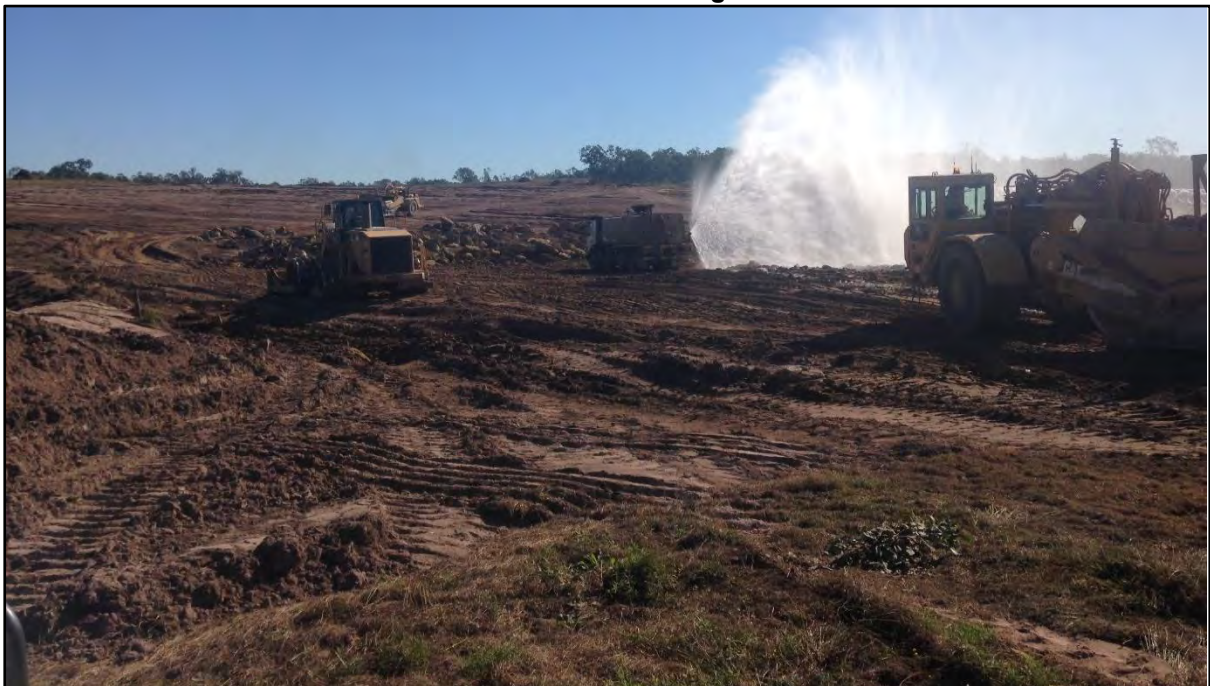
Picture 4: View of the Site During Construction
