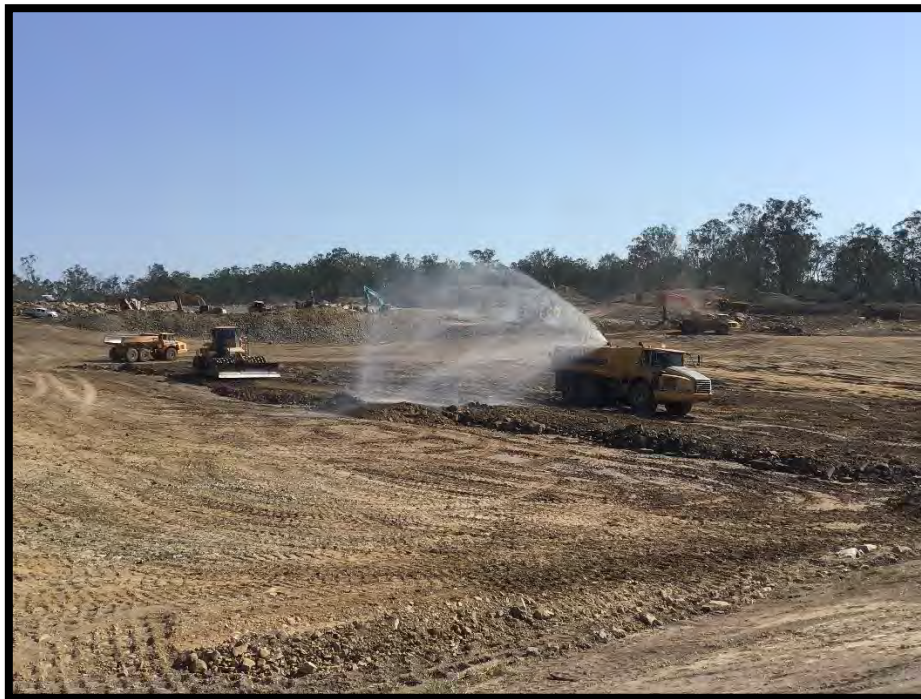
Picture 2: View of the Site During Construction
