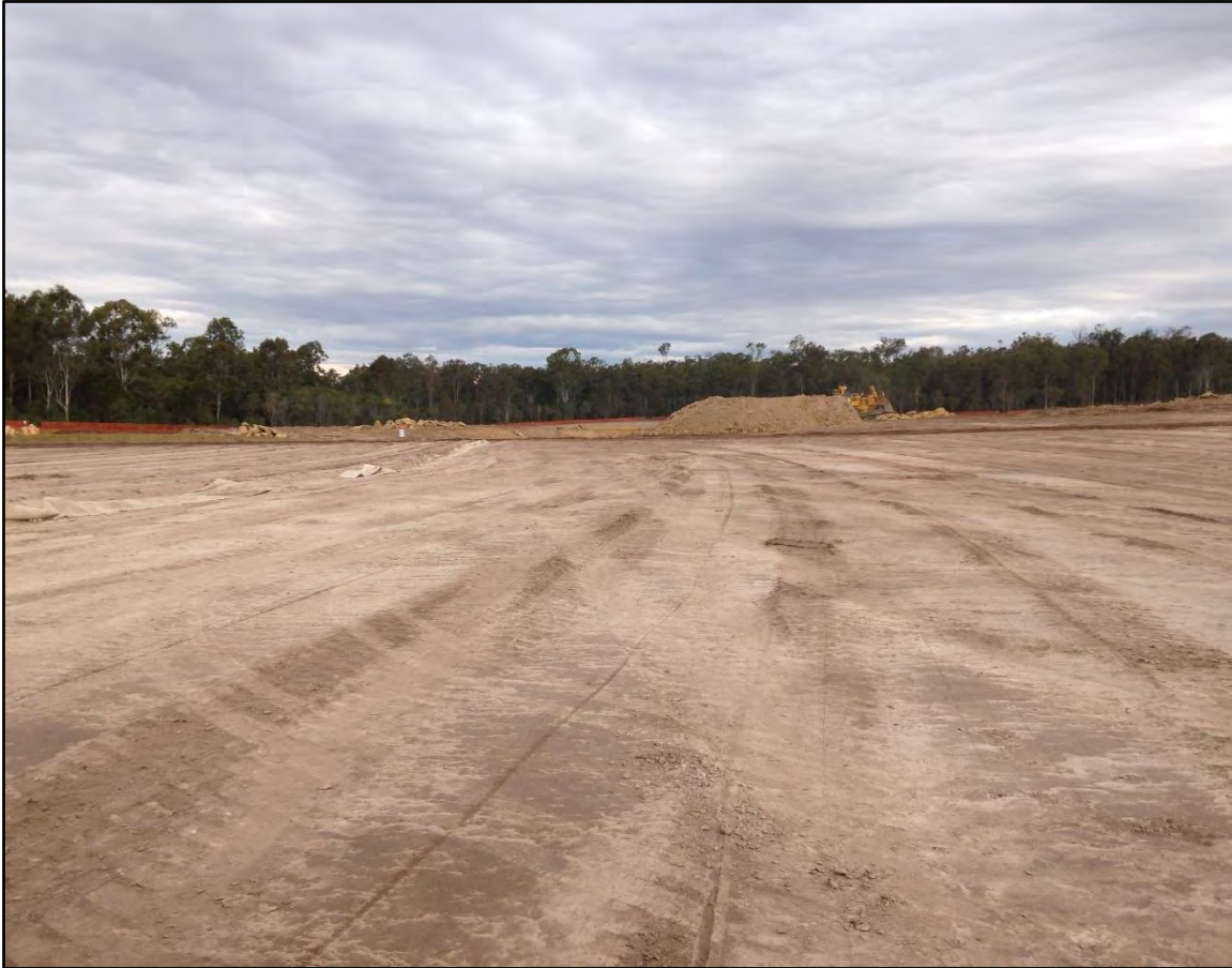
Picture 3: View of the Stripped Surface Prior to Filling Operations
