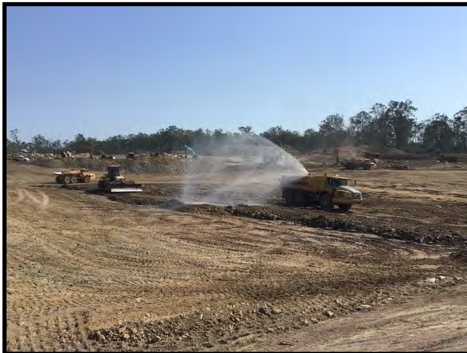
Picture 2: View of the Site During Construction
