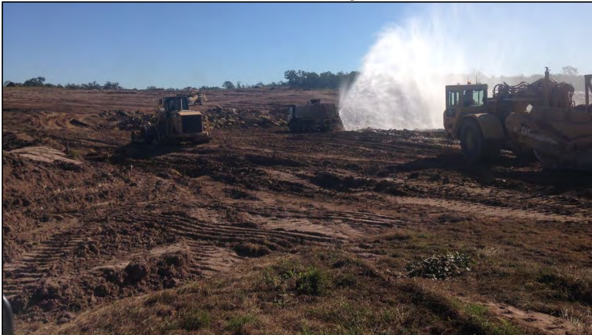
Picture 4: View of the Site During Construction
