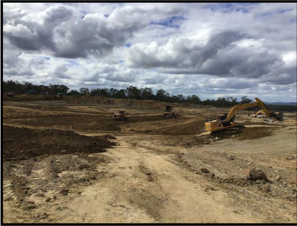
Picture 3: View of the Site During Construction
