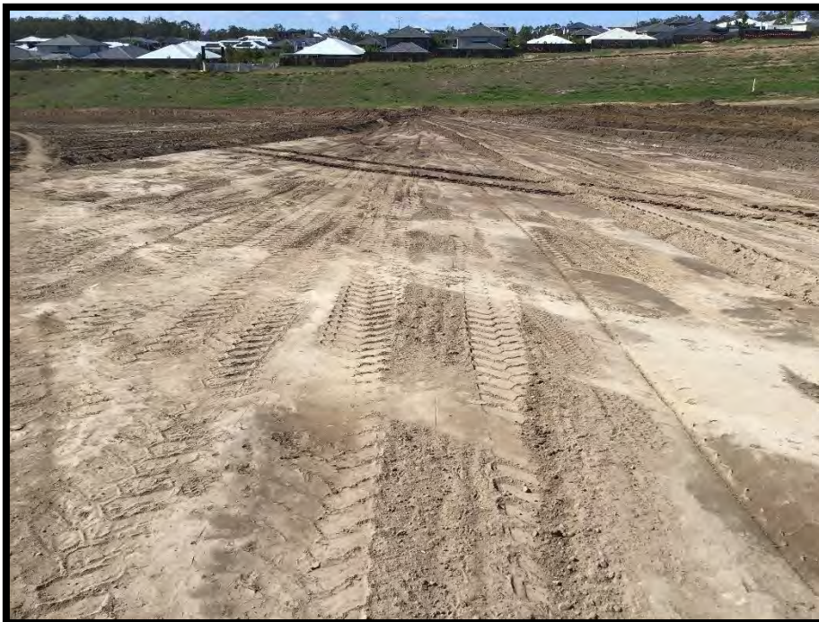
Picture 1: View of The Site During Stripping Operations
