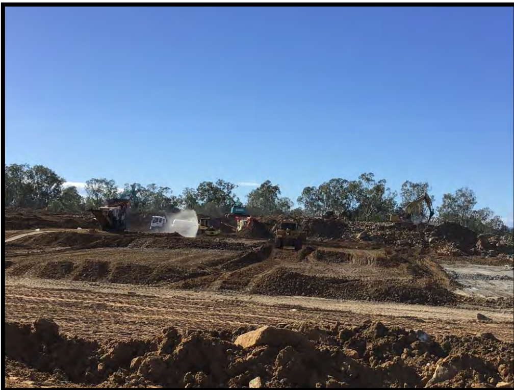
Picture 4: View of the Site During Construction
