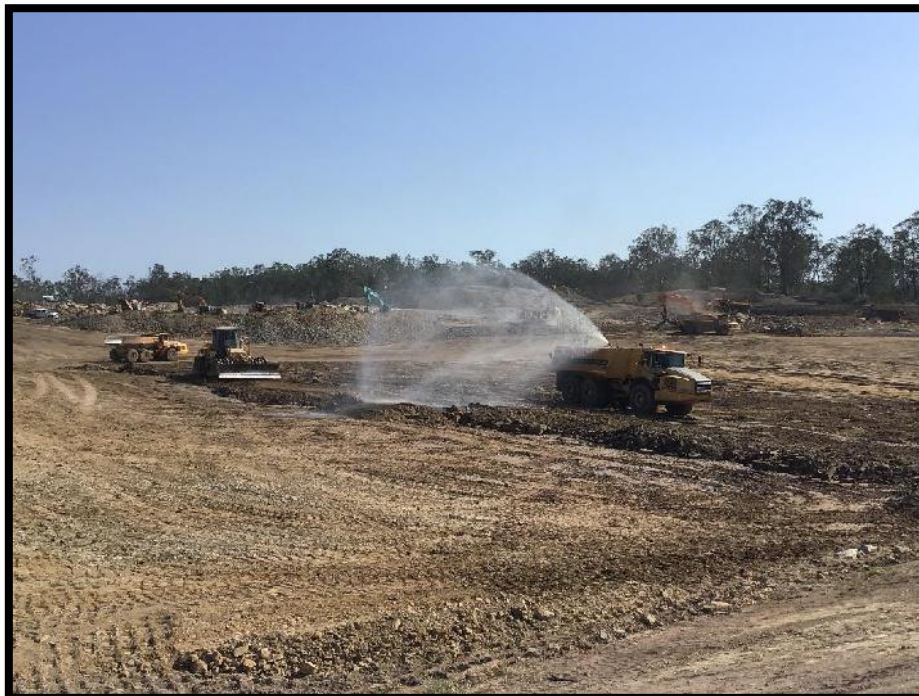
Picture 2: View of the Site During Construction
