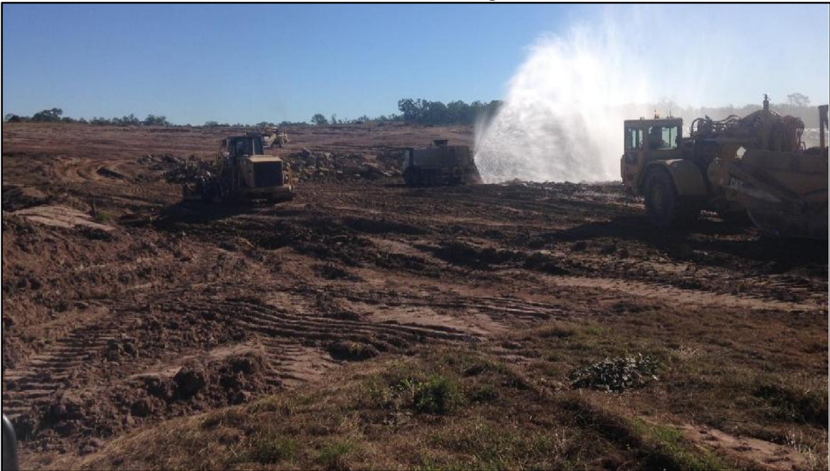
Picture 4: View of the Site During Construction
