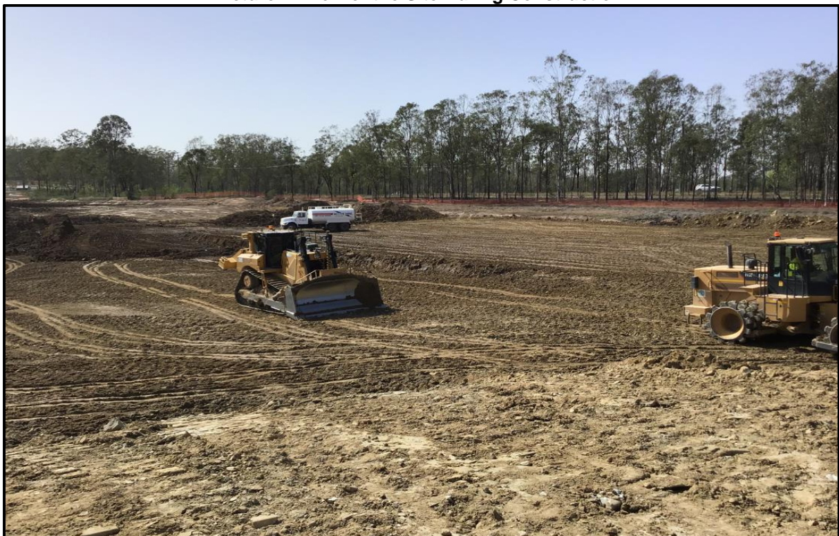
Picture 4: View of the Site During Construction
