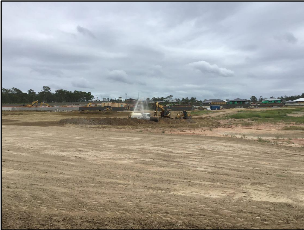
Picture 3: View of the Site During Construction
