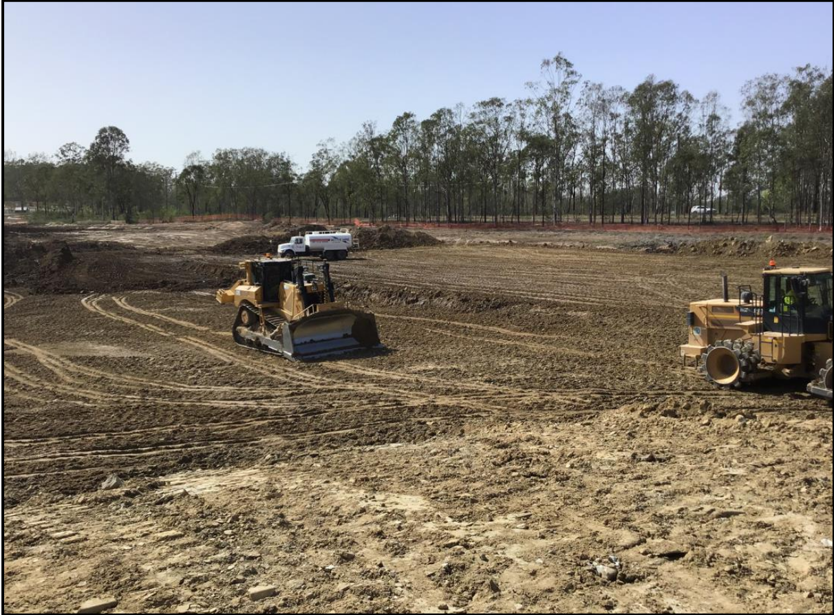
Picture 5: View of the Site During Construction
