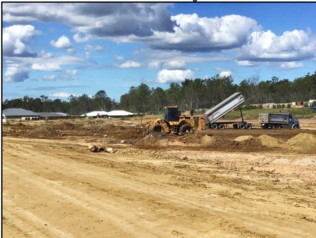
Picture 4: View of the Site during Construction
