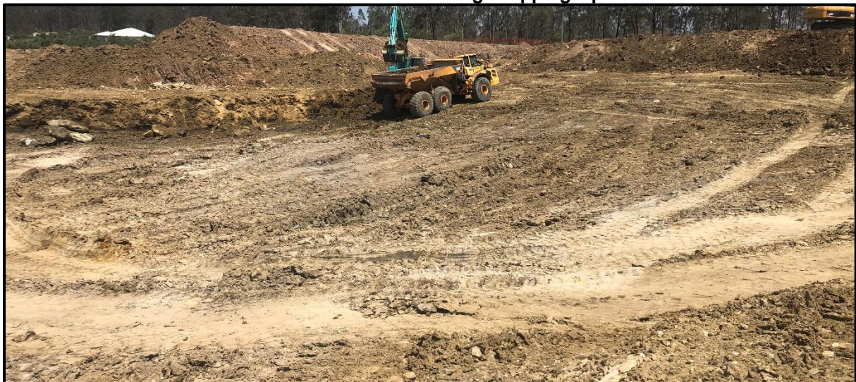
Picture 2: View of The Site During Stripping Operations
