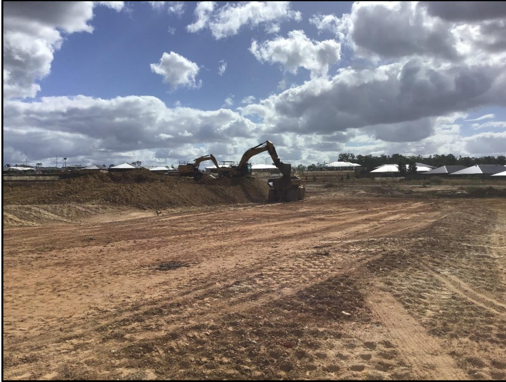
Picture 3: View of the Site During Construction
