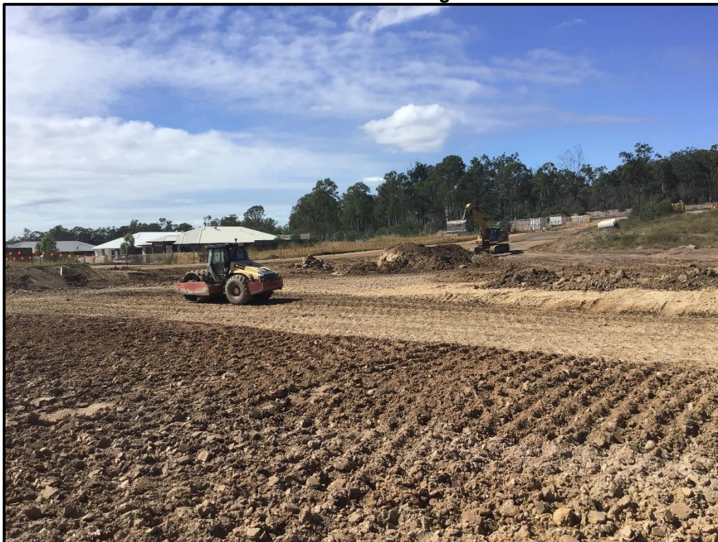
Picture 4: View of the Site during Construction
