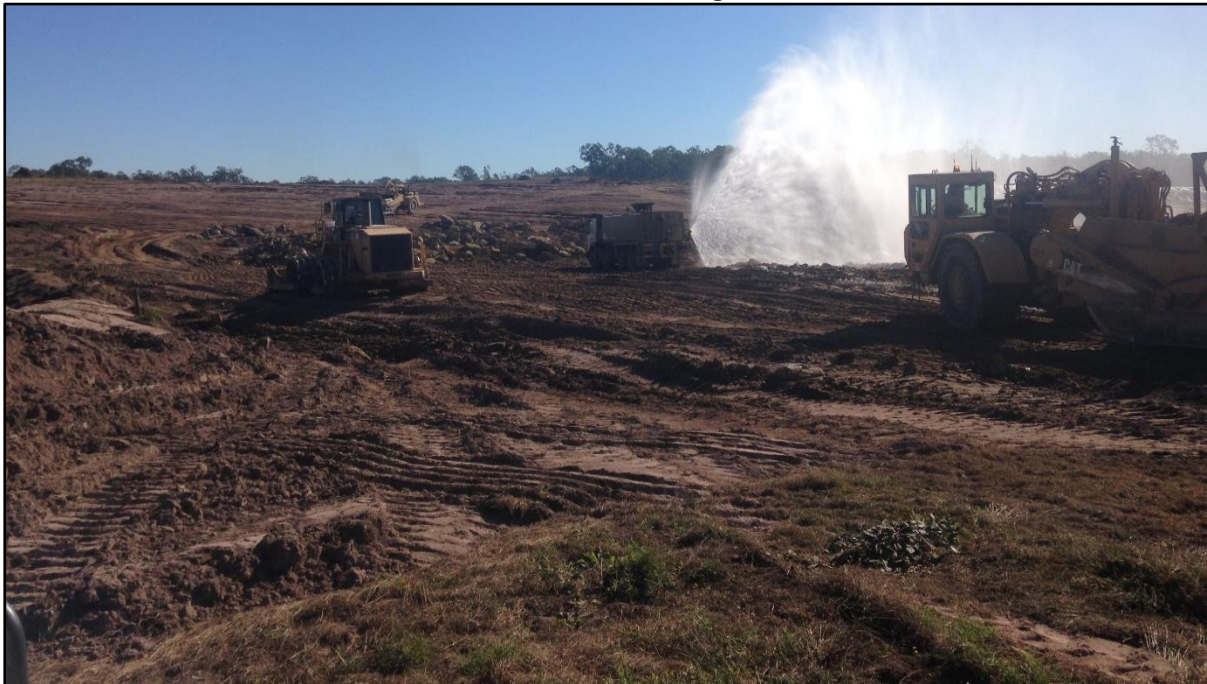
Picture 4: View of the Site During Construction
