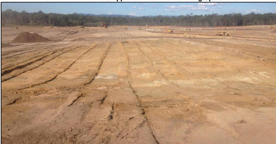
Picture 2: View of the Stripped Surface Prior to Filling Operations
