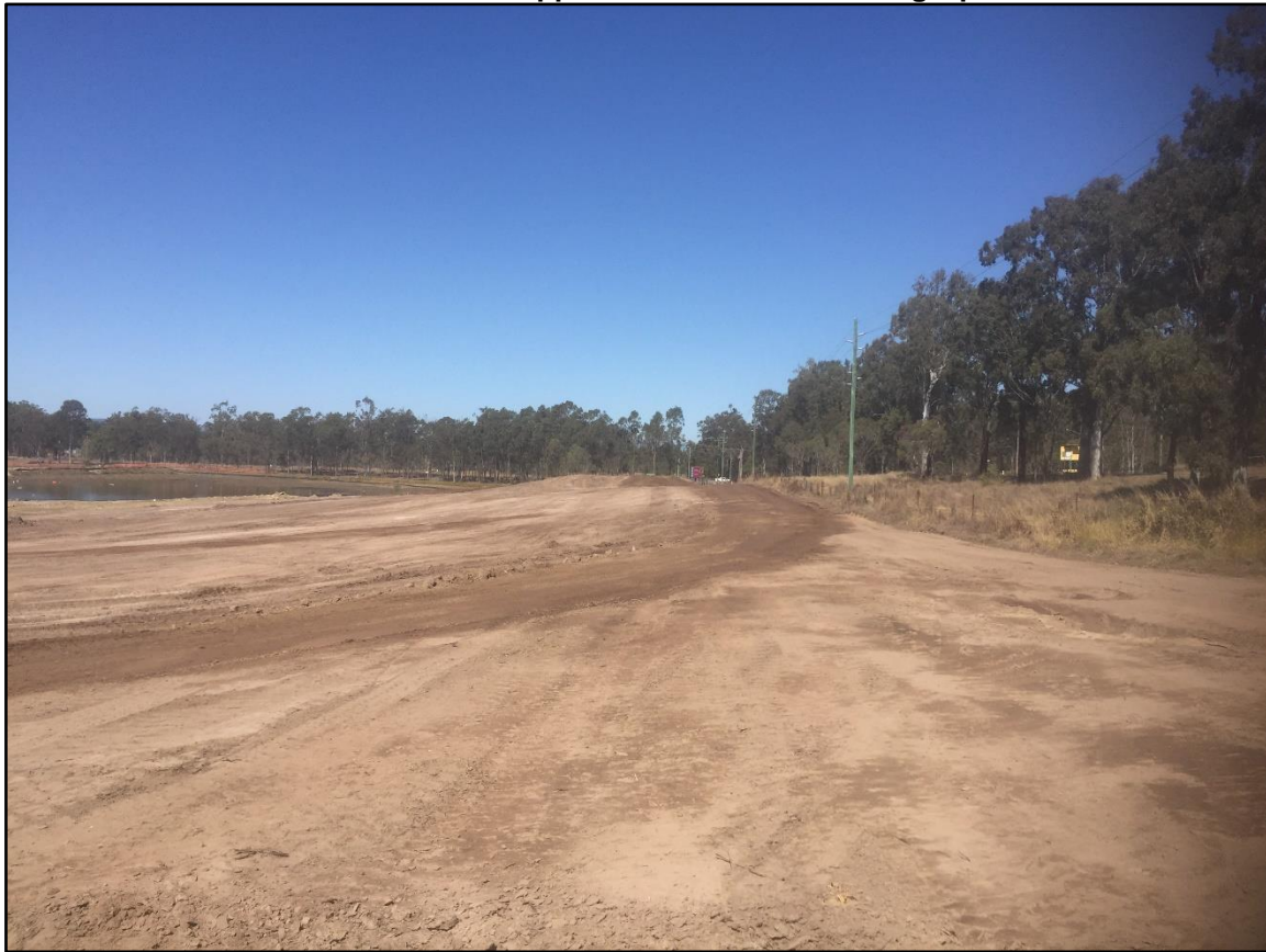
Picture 2: View of the Stripped Surface Prior to Filling Operations
