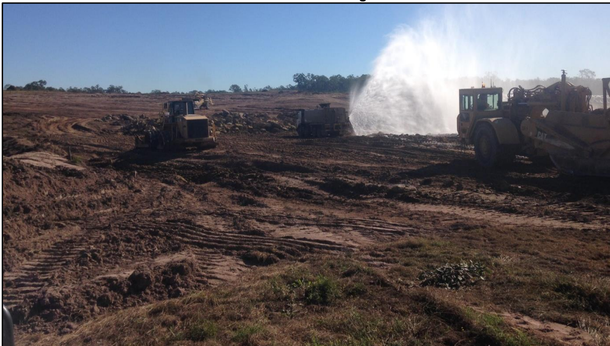
Picture 4: View of the Site During Construction
